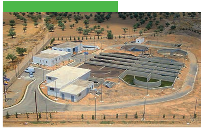
WWTP in Megara, Greece
