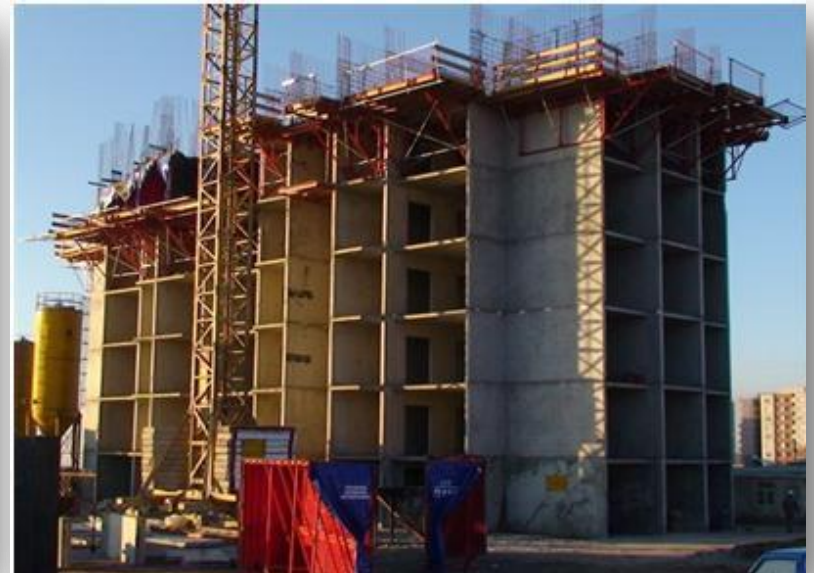
Tunnel formwork system
